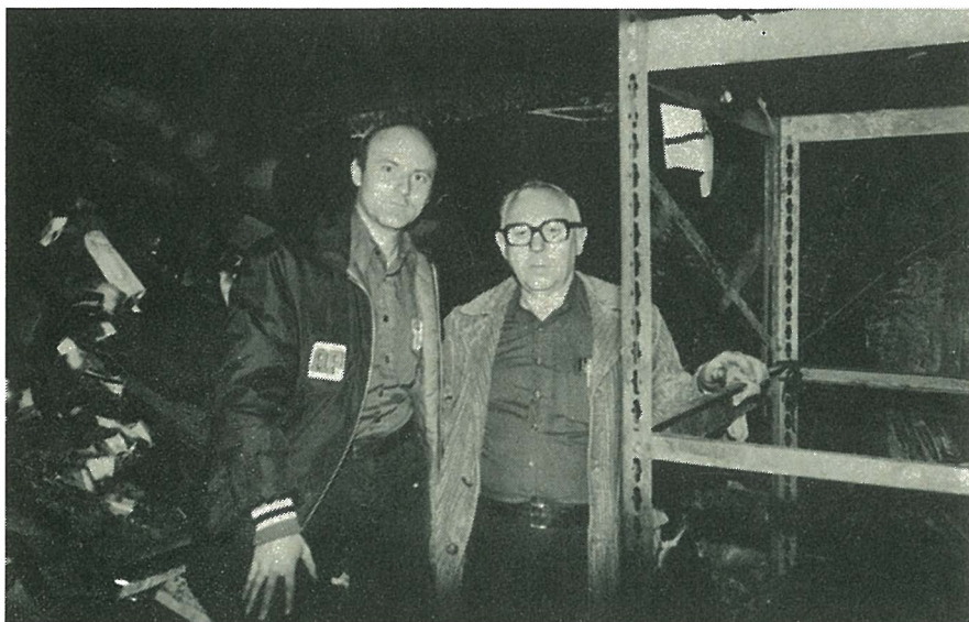
Surrounded by the wreckage of their stock room, Wayne (left) and Wilfred Heimpel look unhappy. But as the old saying goes, 'old soldiers (and jobbers) never die . . .' Both men are determined to carry on.
